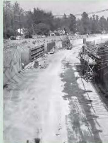
1949: Construction of channel walls for Valley Flood Control Plan
